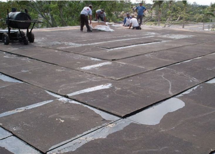
Andrews Roofing LLC installing a 3 ply modified roofing system, Proper installation consist of using proper fasteners, drainage, insulation and ventilation are the key success of a flat roofing system
