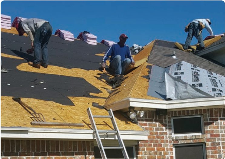
Key success of all roofing system, is using properly trained roofers, preparing the decking, base felt, proper fasteners and spacing, proper exposure, and proper ventilation.
