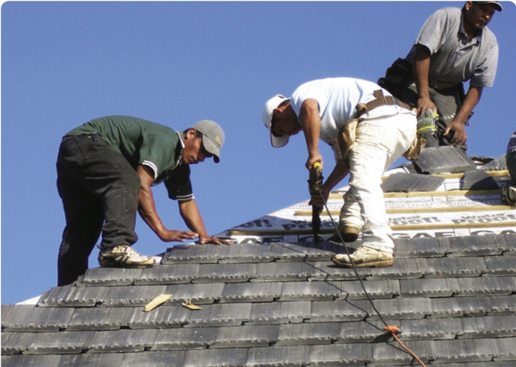
Andrew Roofing LLC installing a flat concrete tile roofing system, Proper installation consist of using proper fasteners, underlayment, batten boards where required, and proper mortar.
